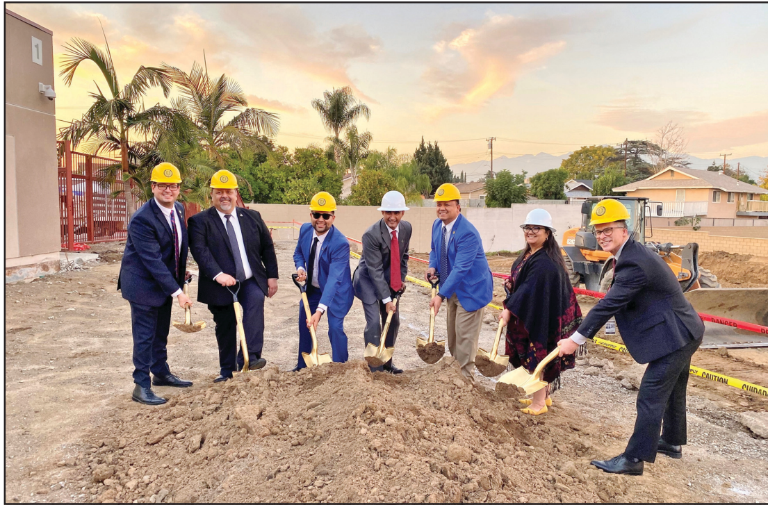
The El Monte Union community came together on Dec. 11 to celebrate the groundbreaking of a new Multipurpose Building and Gymnasium at Fernando R. Ledesma High School. The $13 million facility is being funded primarily by the Measure HS facilities bond. Pictured are Board of Trustees President Florencio F. Briones (left), Board Clerk Carlos G. Salcedo, Member David Diaz, FRLHS Principal Freddy Arteaga, Board Member Ricardo Padilla, Vice President Maria Morgan and Superintendent Dr. Edward Zuniga.
