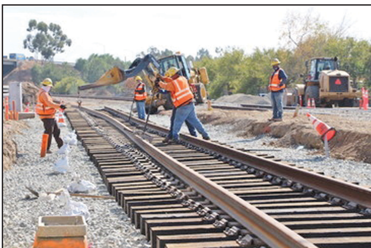
As crews near completion on the Gladstone St. grade crossing in San Dimas, they have begun installing the new track systems - two new light rail tracks (photo 1 left) and one freight track, in its relocated position (photo 2 right).
