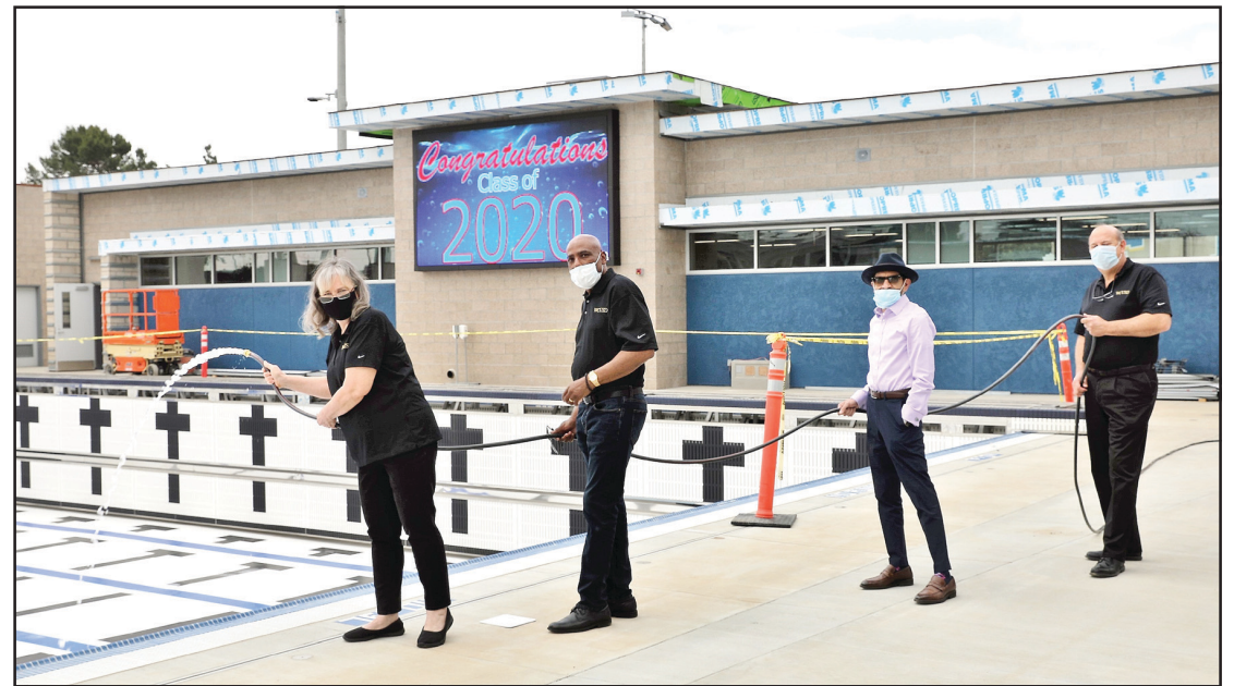
West Covina Unified Board of Education members and Superintendent Dr. Charles D. Hinman begin the pool-filling process at Edgewood High School's new sports complex on May 11. The complex is expected to be completed by July 1.
