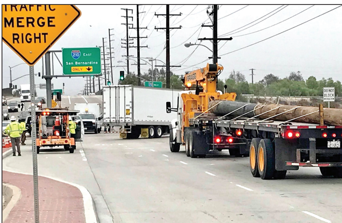
A loaded trailer became detached from a tractor truck striking several Southern California Edison (SCE) utility poles at the intersection of Irwindale Avenue and Camino de la Canterra.
