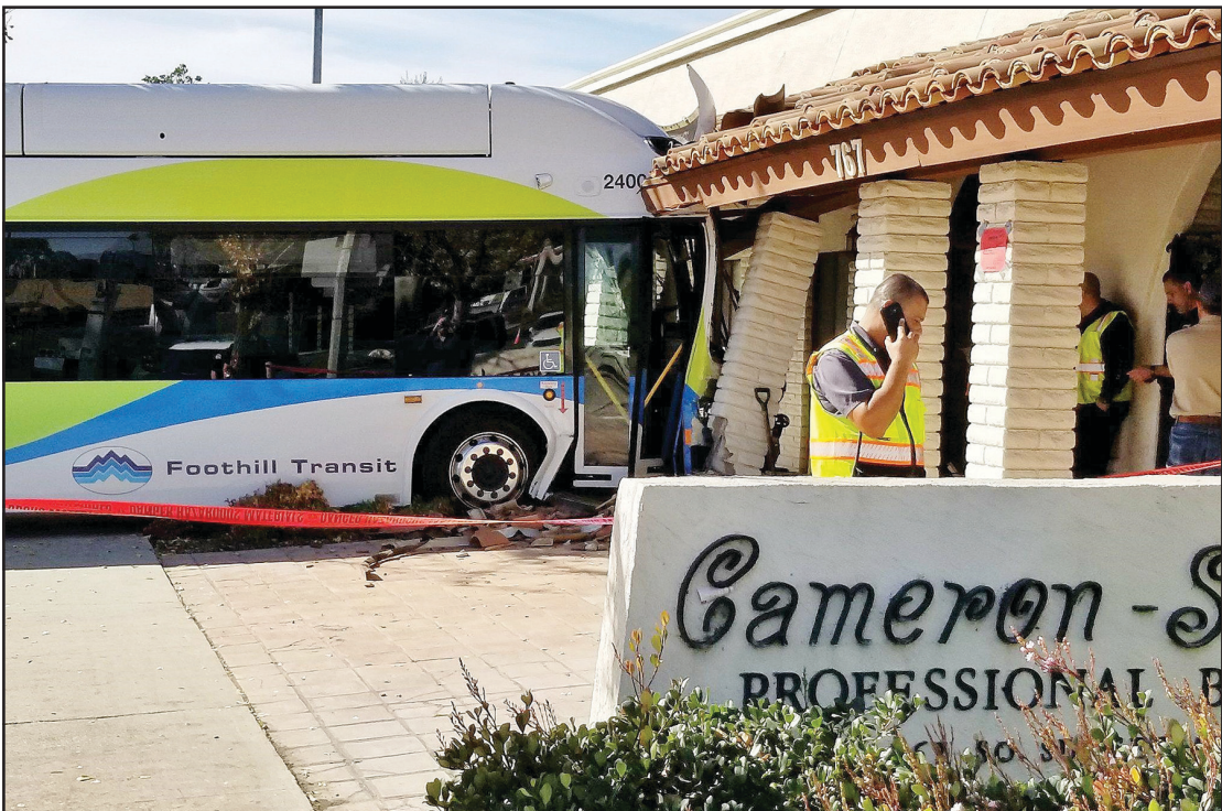
Foothill Transit Bus crashed into a medical building in West Covina.
