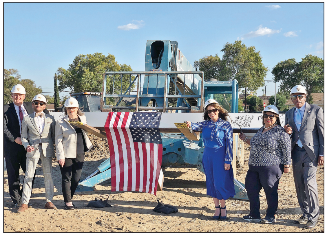
West Covina Unified School District Board of Education members sign their names on a steel beam in a "topping out" ceremony on April 9, celebrating the progress on Edgewood High School's Event Center. Pictured from left to right: Superintendent Charles D. Hinman, Board President Daniel C. Monarrez, Board Vice President Camie Poulos, member Rose Lopez, clerk Eileen Miranda Jimenez and member Michael Flowers.
