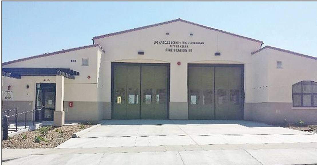
The New, Empty Station 97 completed about five months ago.
