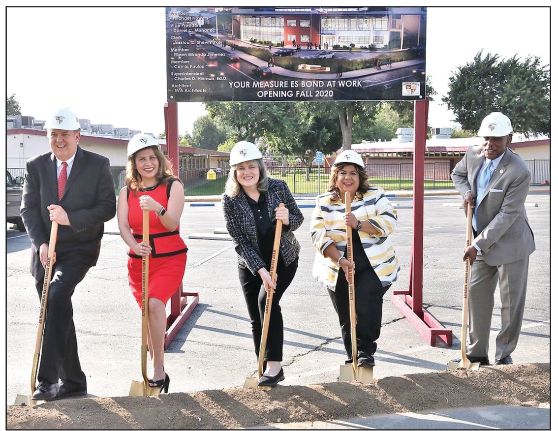
West Covina Unified administrators and Board of Education members break ground on West Covina High School's new science and CTE building on June 25.
