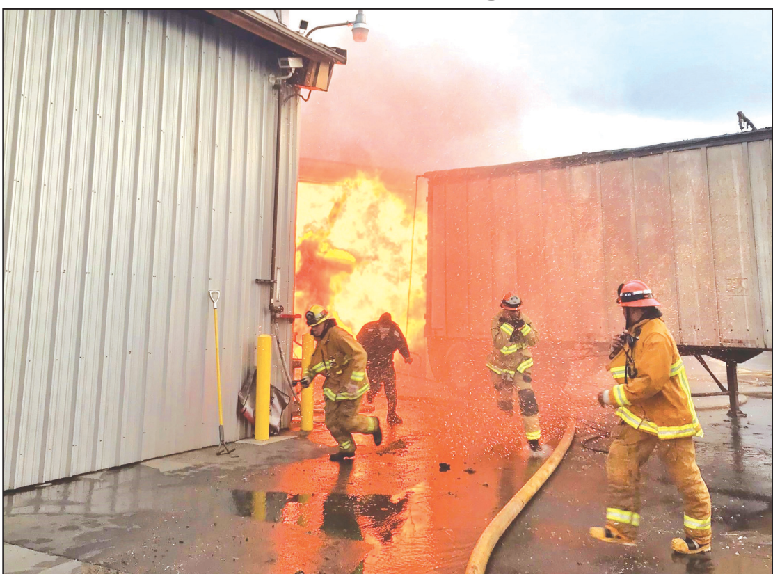
A stubborn fire at a cabinet manufacturing plant got scary when a dust silo exploded into a fireball and sent firefighter running for cover. IPD/L.A. Co. FD
