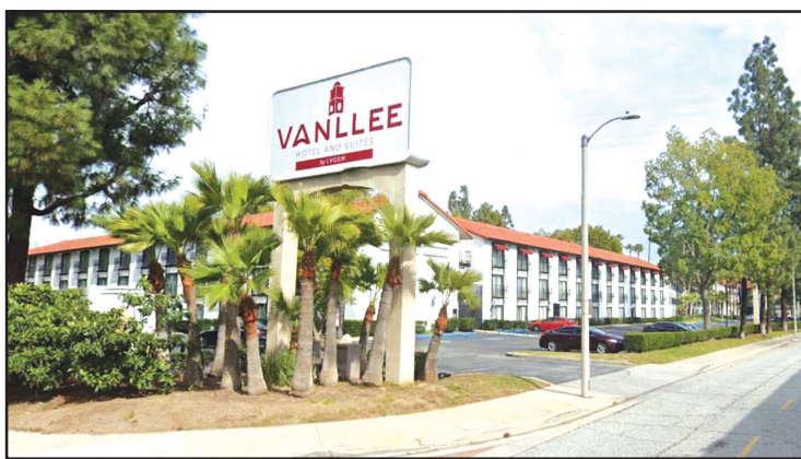
Vanlee Hotel and Suites in Covina will be the site where the homeless and transients will be placed by L.A. County's Project Roomkey.
