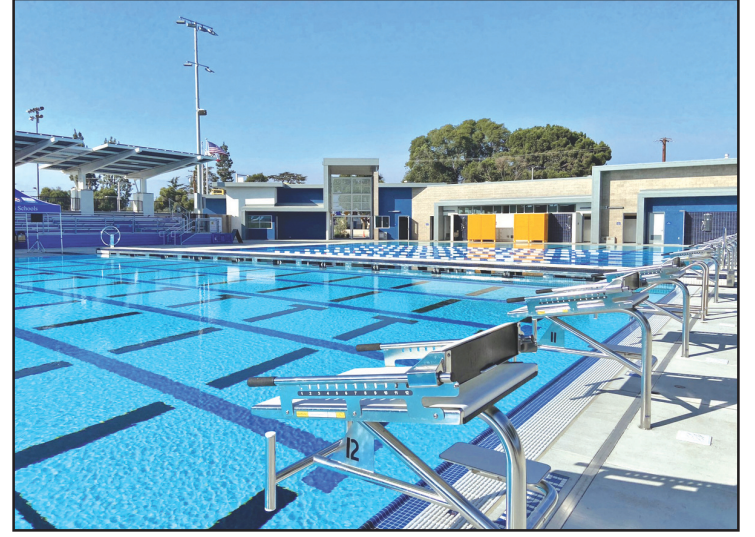
The Olympic-size swimming pool is the centerpiece of the Edgewood Sports Complex, featuring a movable bulkhead to allow multiple activities and competitions to occur simultaneously, thermal shade structures and bleachers.
