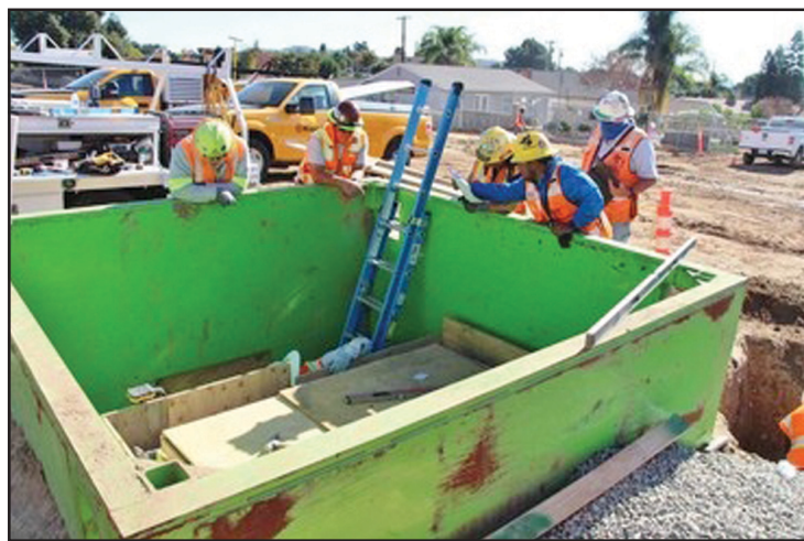
Crews building a storm drain at Barranca Ave.
